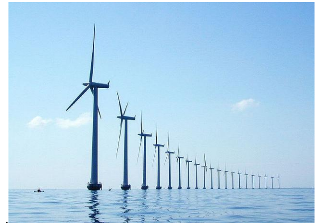
Mads Prahm, Middelgrunden" Offshore Wind Farm, Denmark 2002 (Creative Commons License)
